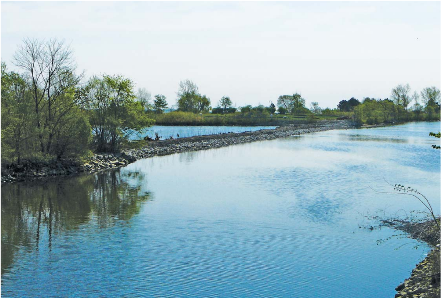
▲ A berm was constructed on the west side of Humber Bay Park East to create a sheltered backwater wetland at the mouth of Mimico Creek.
